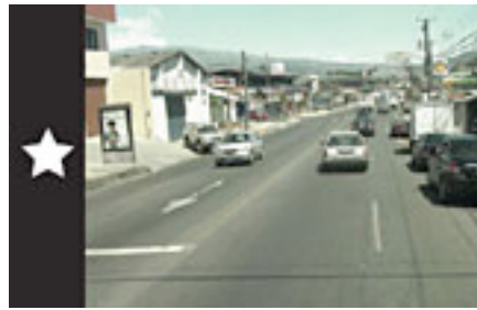
Single carriageway with side friction and roadside obstacles
