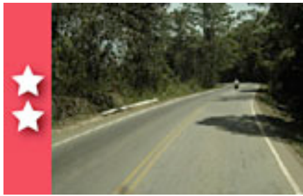
Single carriageway road with sharp curves, narrow paved shoulders and roadside obstacles
